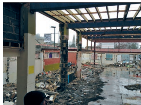
Demolition of the old club almost completed.
